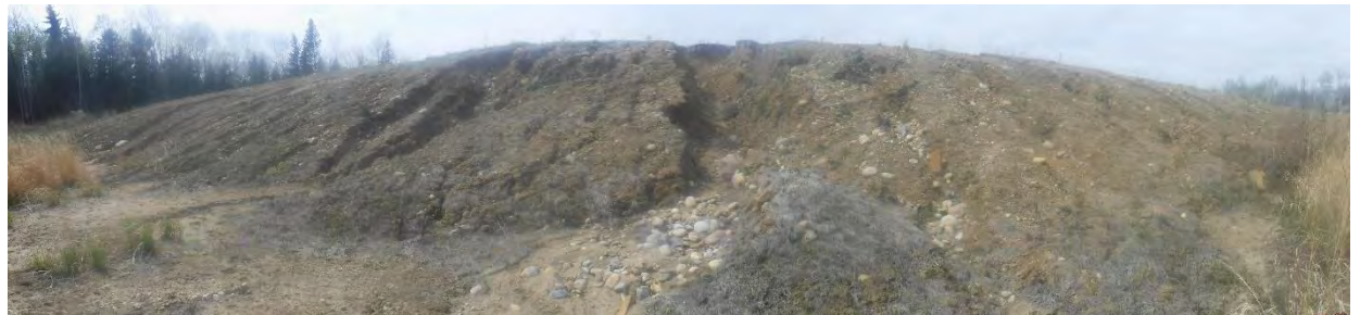
Photo 3: Erosion along the south boundary
