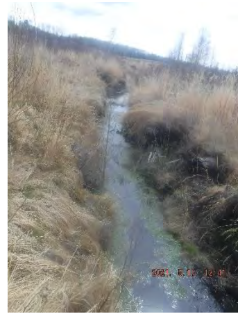
Photo 6: Ditch looking north, slumping along ditch.
