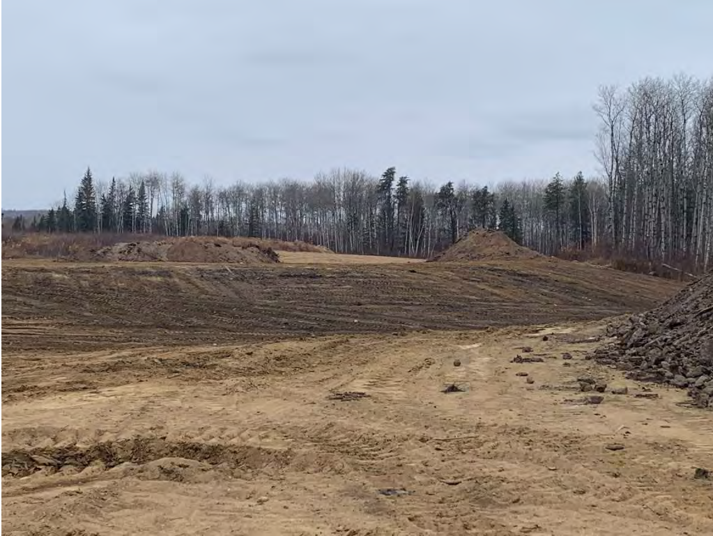
Photo 1: Photo taken looking North at the low-lying area where all the buried topsoil and woody debris was salvaged.
